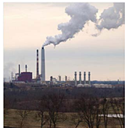
Test Facility for 0.7 MWe Slipstream Study
