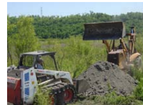
Excavating ash for processing
