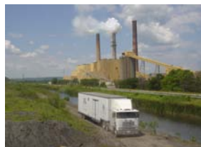
Moving plant to site
