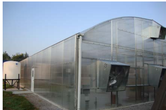
Figure 2. 2700 sq ft greenhouse containing photobioreactors
