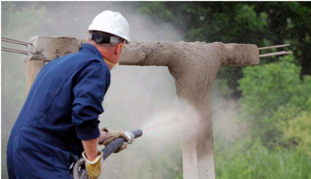
A researcher uses a hose to spray Tekcrete Fast™ onto the joint of a beam.
