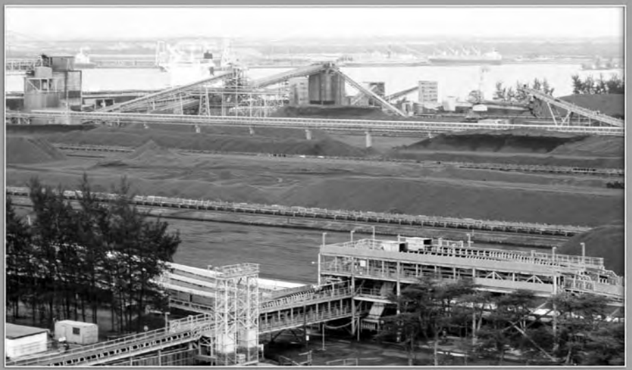
Richards Bay Coal Terminal
